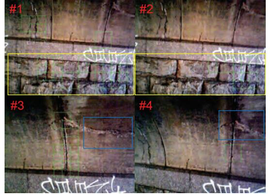
Fig. 9. The over detection and missed detection cases in field test 1. The orange rectangles denote over detection, and the missed detection are represented with blue rectangles.
