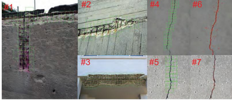
Fig. 5. Results generated by our deep based detection model with CSSC database, where the green rectangle denotes the region of spalling and crack. In images #6 and #7, the red features denote the post-labeling of the crack for evaluation, where the width of the crack can be achieved via stereo-vision.
